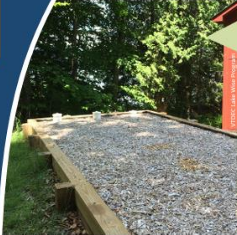
Alternative bottomless sand filter dispersal system.
