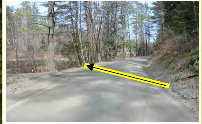
New Culvert Location
