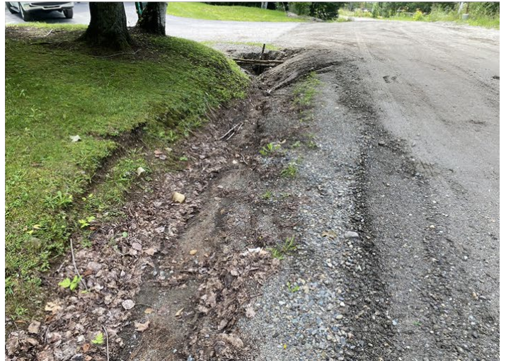
Figure 20. Common issues observed in the watershed were unstable ditches and uncompacted ditch slopes leading to sediment transport.
