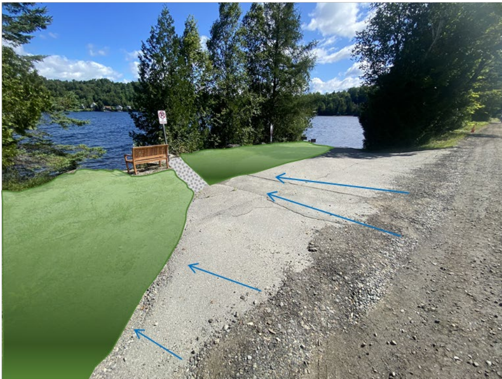
Figure 17. Currently, stormwater flows pass over loose sparsely vegetated shoreline before entering Shadow Lake (upper). It is recommended that this area is vegetated with native species per the VT Bioengineering Manual (VT DEC, 2022) to stabilize the shoreline and filter stormwater (conceptual retrofit is shown overlaid in lower photo).
