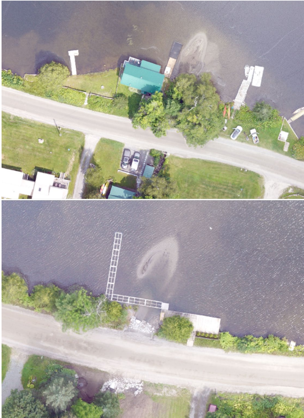
Figure 35. Significant sediment was deposited in Shadow Lake from stream culverts following the July 2023 storm event.
