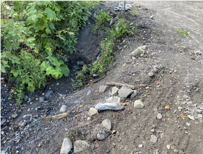
Figure 20. Common issues observed in the watershed were unstable ditches and uncompacted ditch slopes leading to sediment transport.
