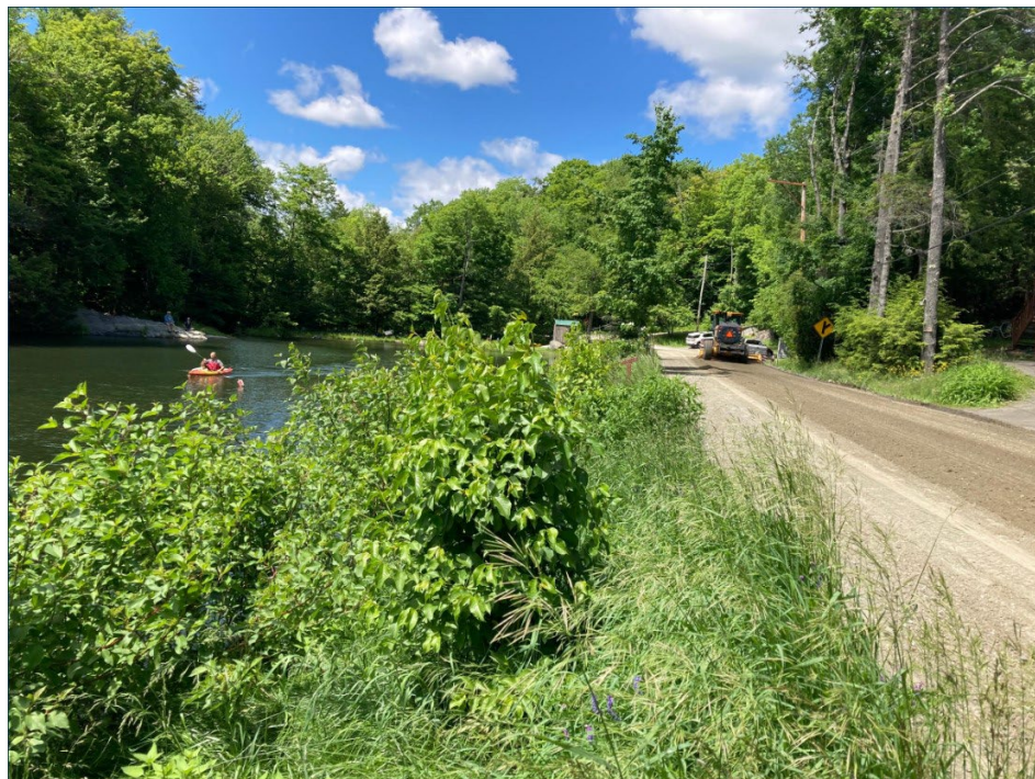
Figure 43. An example of a bioengineering project, encapsulated soil lifts, on Lake Raponda in Wilmington, VT (Source: VT DEC Lakes and Ponds). Prior to the installation this project, the road bordering the lake was eroding, the lakeshore was narrow and steep, and the road was being undercut causing sediment and pollutants to enter the lake.
