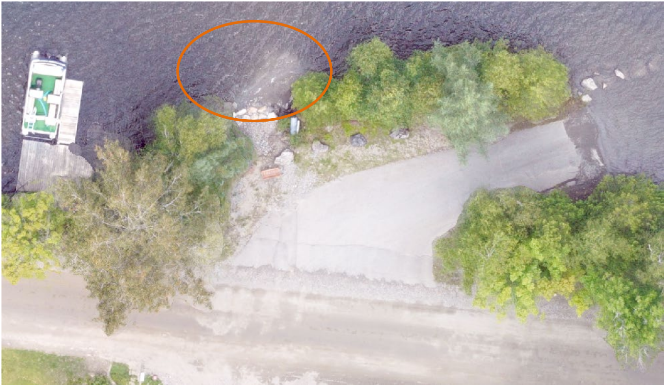
Figure 16. Sediment deposition can be observed adjacent to the boat launch area (see area highlighted by an orange circle).
