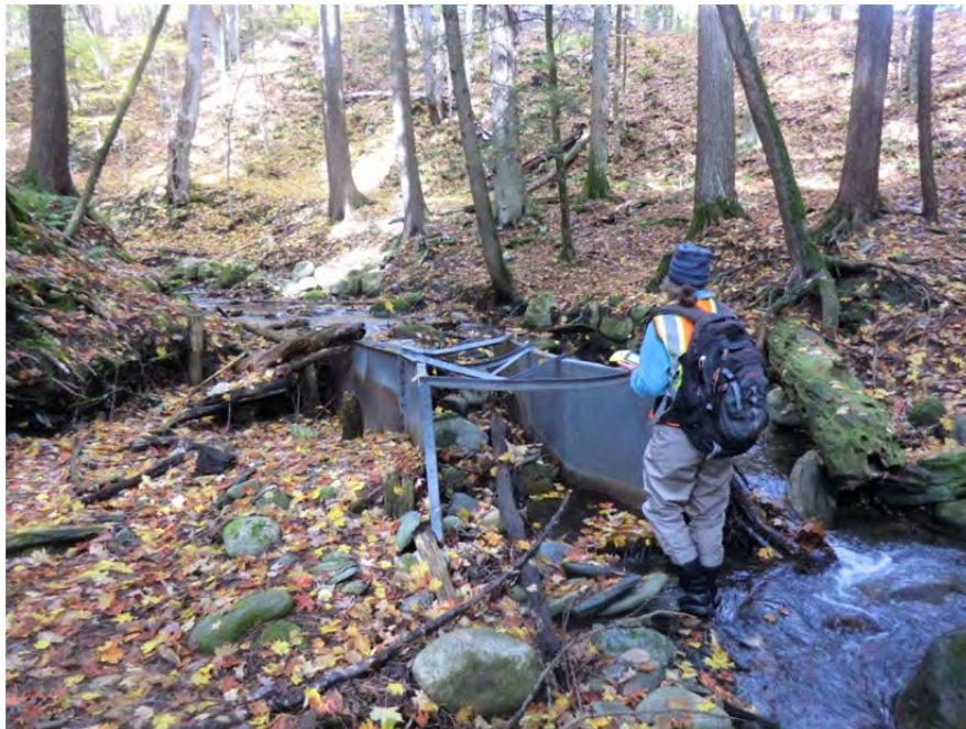
Figure 22. Remnants of Parshall Flume Stream Gauging Structure
