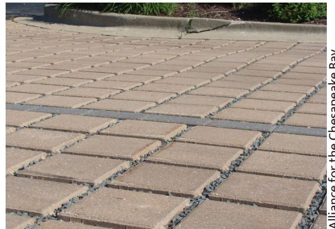
Clockwise from top left: geogrid reinforced peastone, turf block pavers, block pavers
