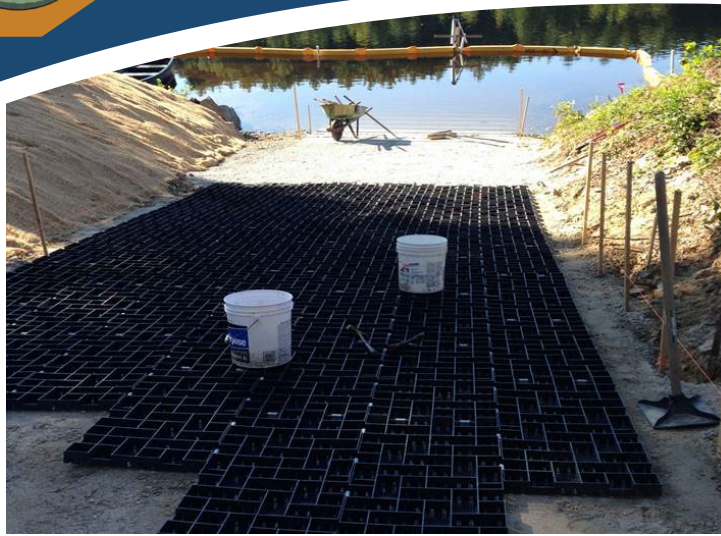
Geogrid boat ramp for erosion control infiltrates rainfall at the source and protects water quality.
