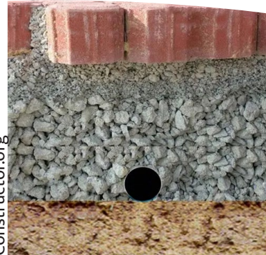
Layers of pavers and stone.
