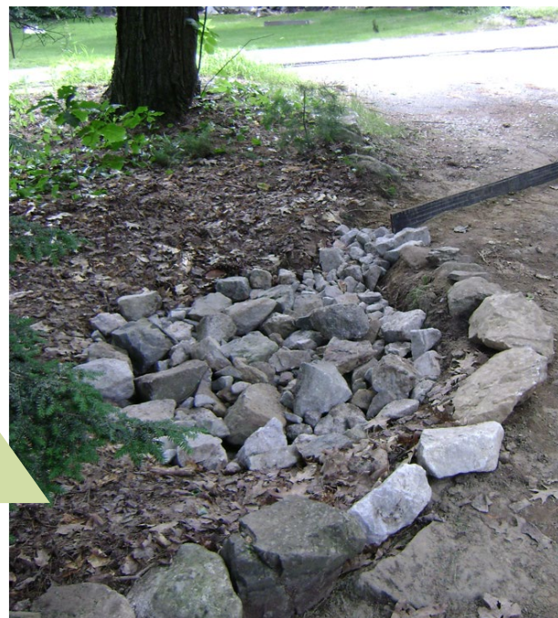
A dry well receives driveway runoff.
