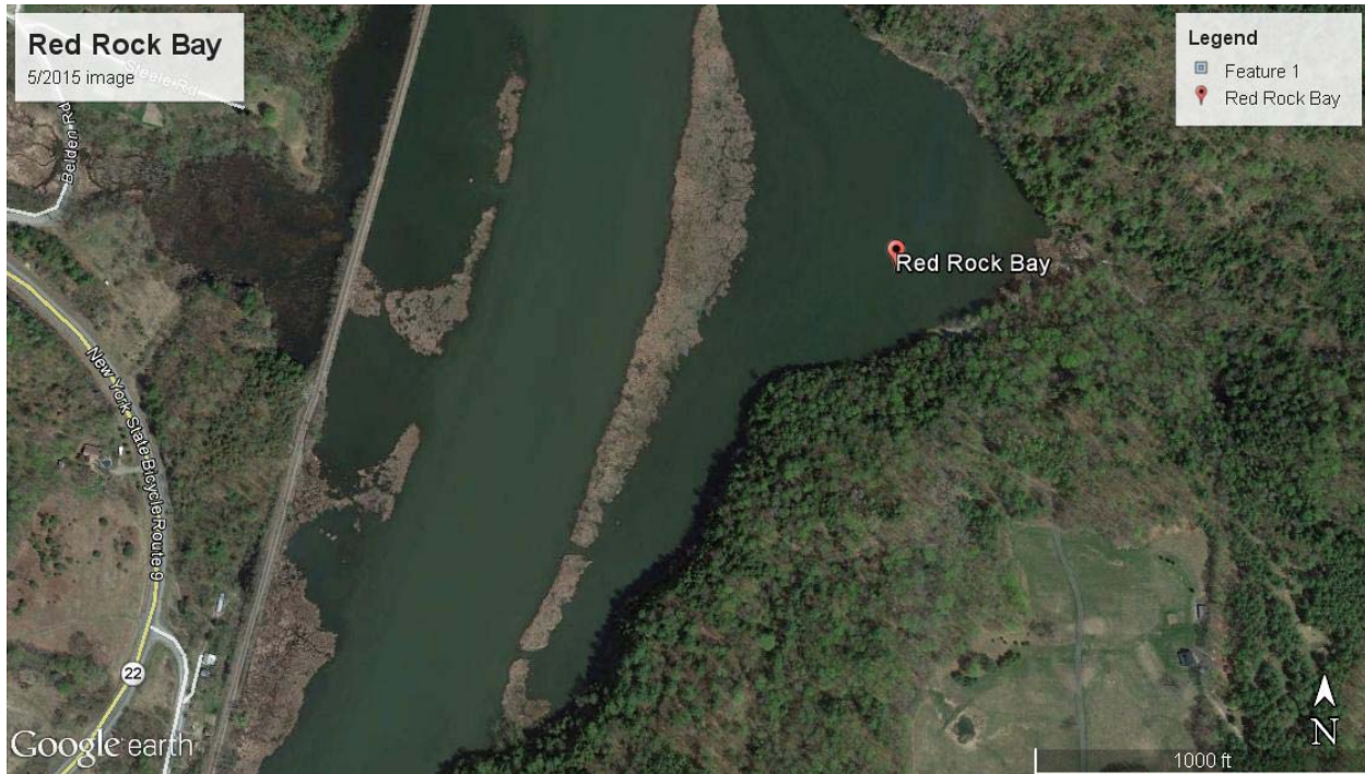
Channel at south end of Red Rock Bay under low water conditions in May 2015. The southernmost opening is the channel where widening is proposed.
