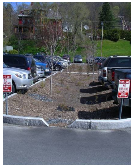
INFILTRATION TRENCH IN A MONTEPELIER PARKING LOT
