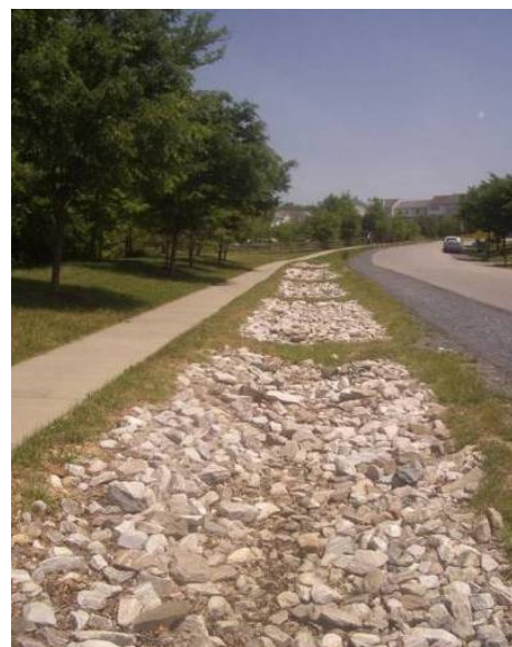
ROADSIDE INFILTRATION TRENCH
