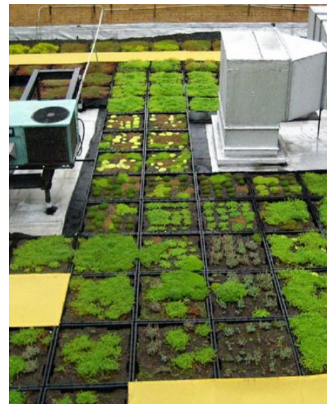
EXTENSIVE GREEN ROOF, NEW YORK
