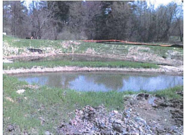
STORMWATER DETENTION POND
