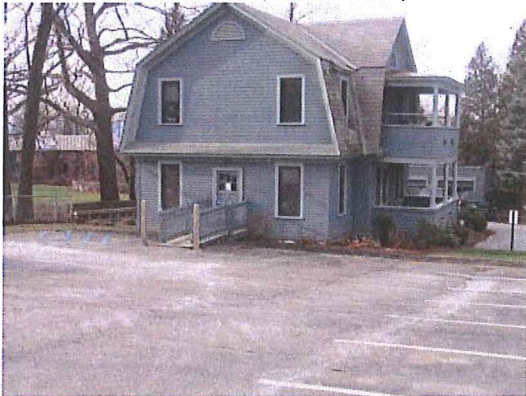
West house (wet basement at times)
