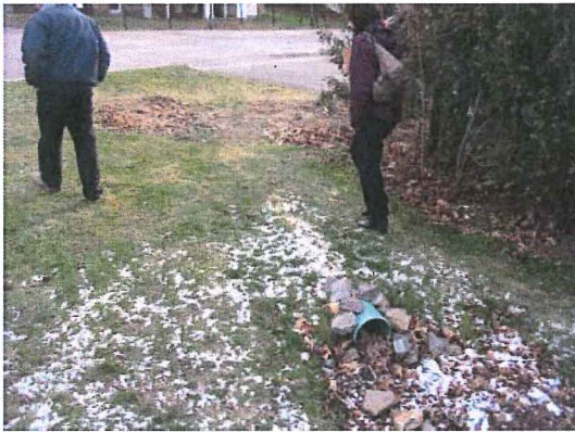
Discharge pipe to stone drainage swale
