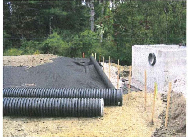
INFILTRATORS WITH TANK
