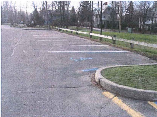
Runoff leaves parking lot (no curb) and continues toward Coolidge House
