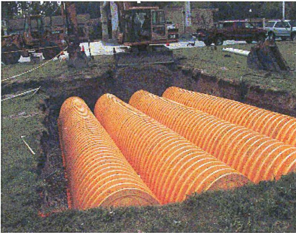
INFILTRATORS IN LAWN AREA
