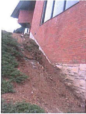
Slope beside Hauke Family Campus Center: Rooftop runoff/foot traffic causing erosion of slope
