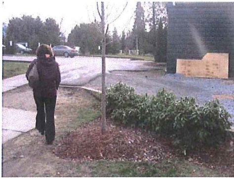
Area near Carriage House Poorly graded area
