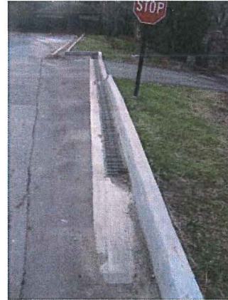
Trench drain collecting runoff to discharge into stone drainage swale
