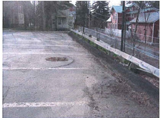
CB grate filled in with leaves
