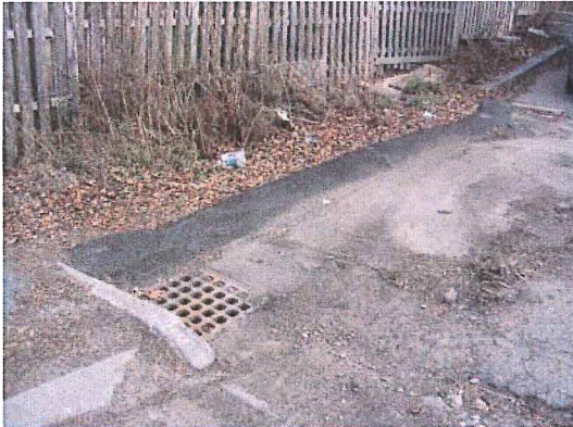
Catch basin at end of Harrington Terrace
