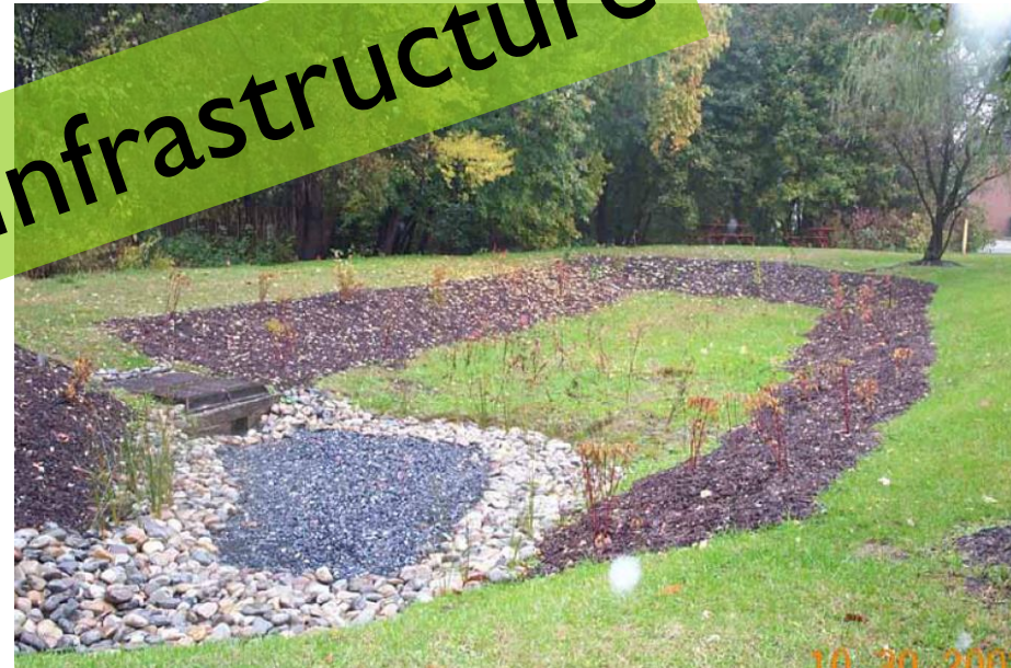
Detention Basin After Retrofit with Water Quality Enhancements
