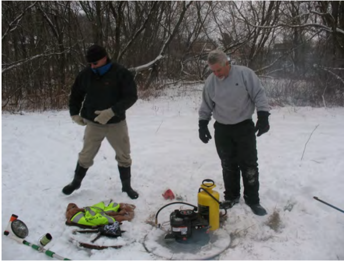
Figure 9. Smoke testing at sewer manhole SMH#9-A (near Willow Street)
