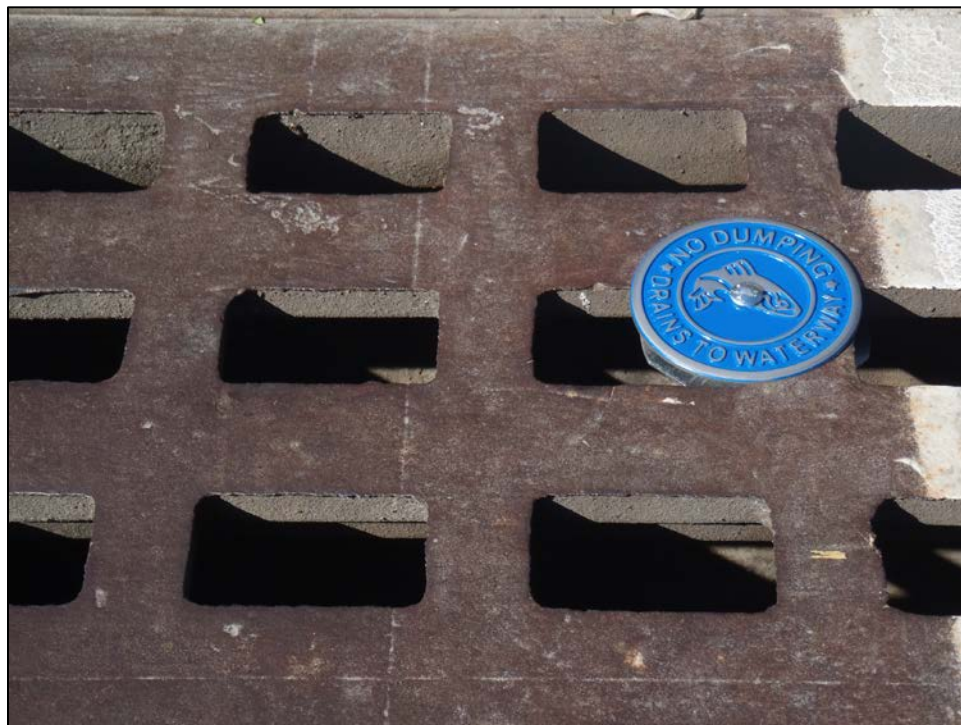
Figure 8. Catchbasin grate (CB-B) with "No Dumping" placard
