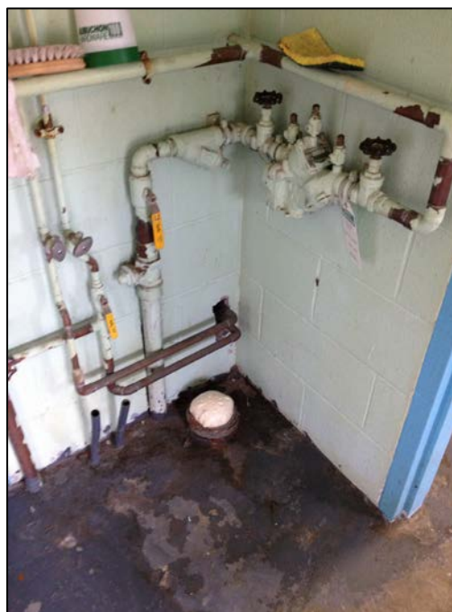
Figure 2. Sealed utility sink drain
