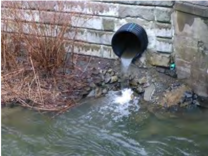
Figure 1. Typical stormwater system outfall after a rainstorm.
