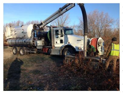
On November 25, 2013, Hartigan televised the trunkline with the assistance of the City. Video logs of the camera inspection and a report by Hartigan can be found in Appendix G. Hartigan approached the trunkline from three (3) different directions. The first began in back of SB Collins near the old CVPS cooling ponds. Hartigan began televising upstream of TL-8 towards the Briarwoods Trailer Park. The camera inspection went a total distance of 140' before it encountered an underground
