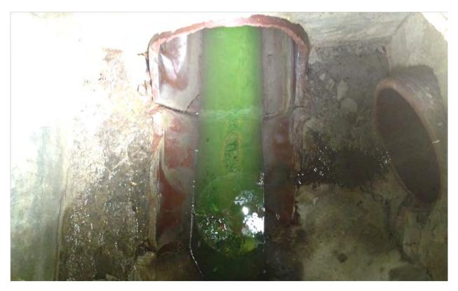
Dye testing of toilets in two houses on North Pleasant Street in Middlebury revealed cross connections to a stormwater line, visible in this manhole above
