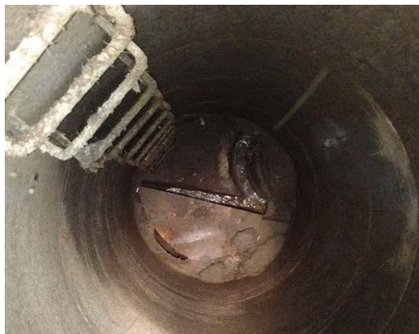
Figure 2: Sanitary manhole sump prior to repair.
