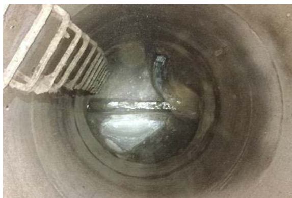
Figure 1: Sanitary manhole sump after repair. Note grout blocking pipe inlet.
