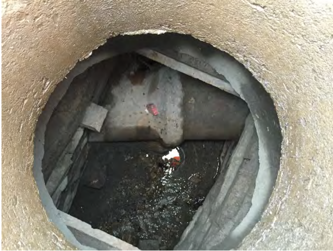
Figure 2. Stormwater manhole MH1 with concrete sewer main running through it
