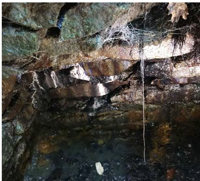
Figure 3. Interior face of CB4 showing wastewater infiltration
