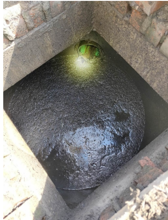
Figure 20. Dark, muddy water in catchbasin CB02
