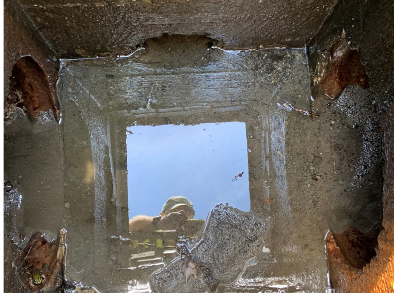
Figure 11. Pipe junctions in catchbasin CB01
