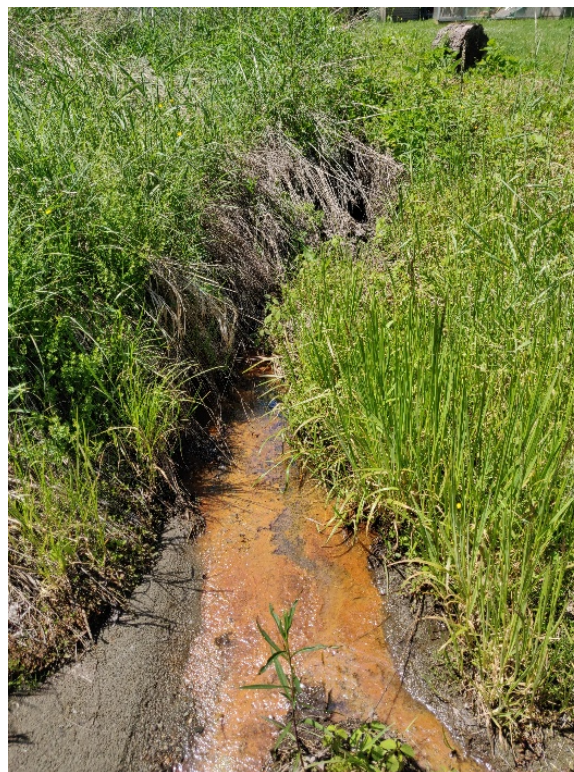
Figure 5. Iron staining in swale below outfall CT01
