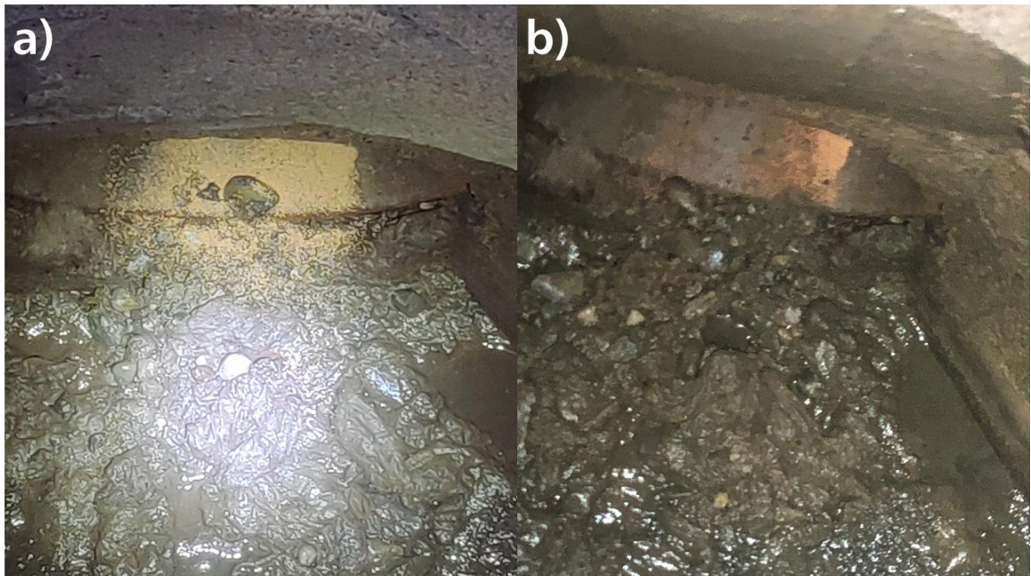
Figure 18. Manhole MO01-MH1: a) Cork placed in inlet pipe; b) after flow on August 17, 2020
