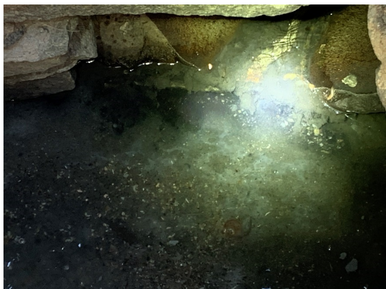
Figure 3. Biofilm indicating wastewater contamination in MH11
