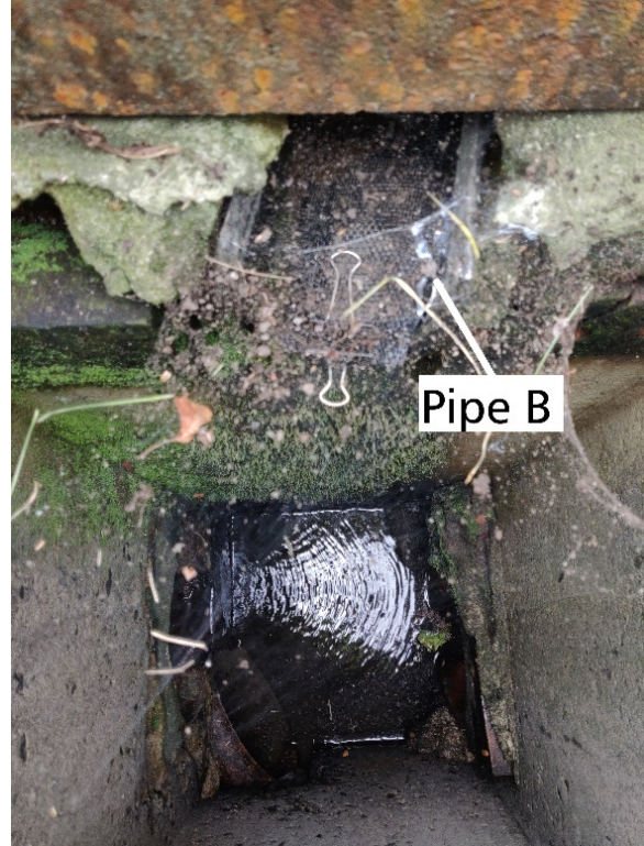
Figure 16. Unmapped pipe enters catchbasin CB28
