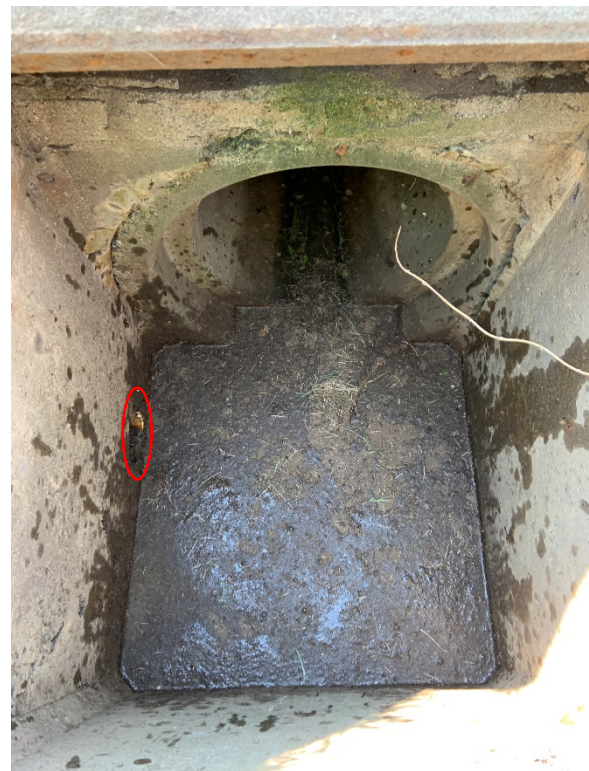
Figure 21. Pipe (circled) entering catchbasin CB1
