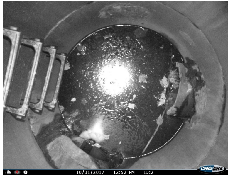
Figure 15. Detergent suds entering manhole CB7
