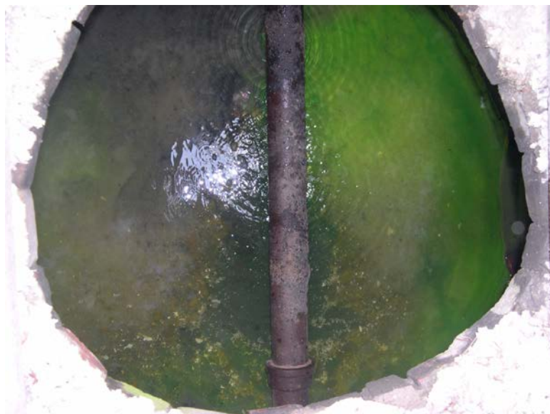
Photo 3. Catch basin BR-920C. Note green dye from sewer system
