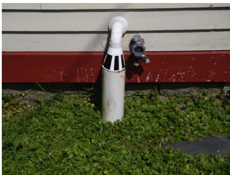
Photo 1. Outlet of sump pump in system discharging at BR-800
