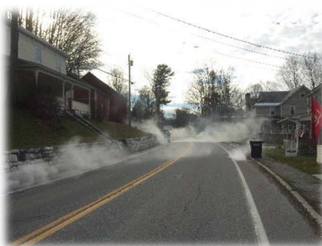
Smoke testing PWL-19 in Pawlet.
