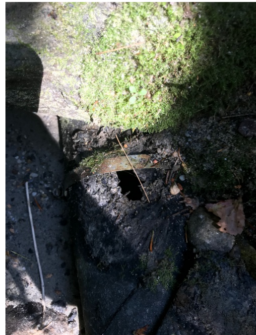
Figure 5: Broken sewer lateral in catchbasin CB1
