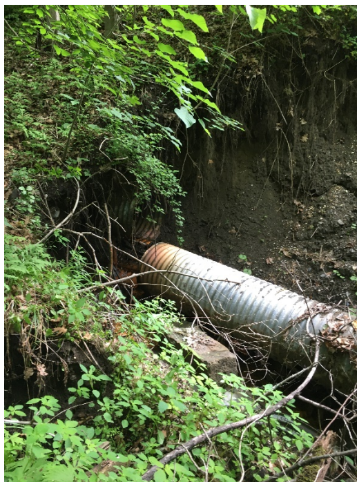
Figure 3. Broken stormwater outfall and significant erosion around PU240
