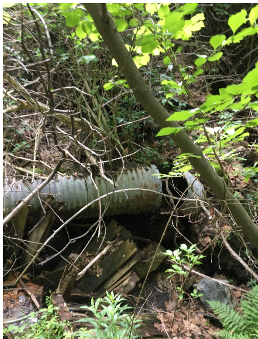
Figure 2. Erosion and broken stormwater pipes in the gulley containing PU230 and PU240
