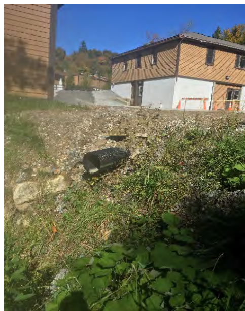
Figure 7. Newly constructed outfall adjacent to 75 Okemo Ridge Road
