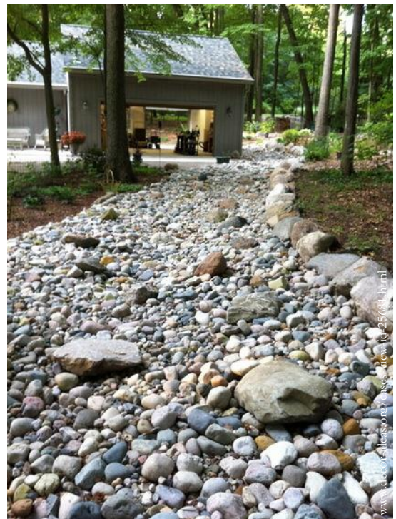
Infiltration trenches can be a practically invisible part of a lawn, or they can be topped with decorative stone as a landscape element.
