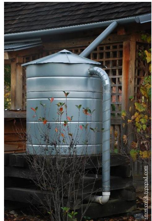
Cistern storing water on a residential property.
