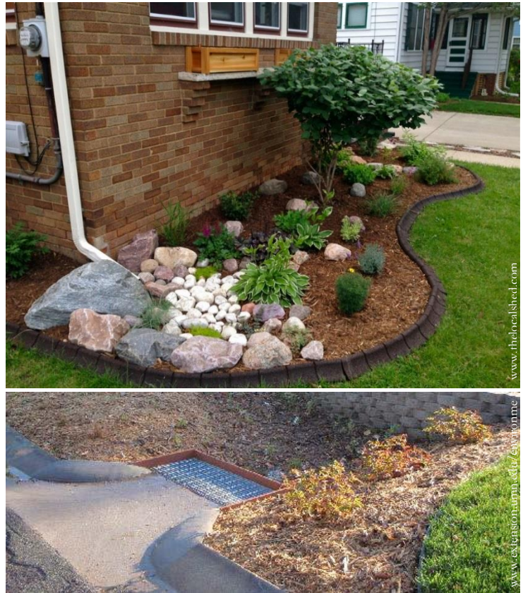
Top: Rooftop runoff can flow directly into rain gardens, though you may need a splash pad or some stone to slow the water down. Bottom: Bioretention areas that are larger or treating runoff from areas with higher sediment loads need some pre-treatment (like this “Rain Guardian”) to settle out sediment and debris.
