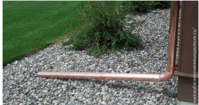
Downspout disconnection to a residential lawn, with gravel bed to evenly distribute runoff.
