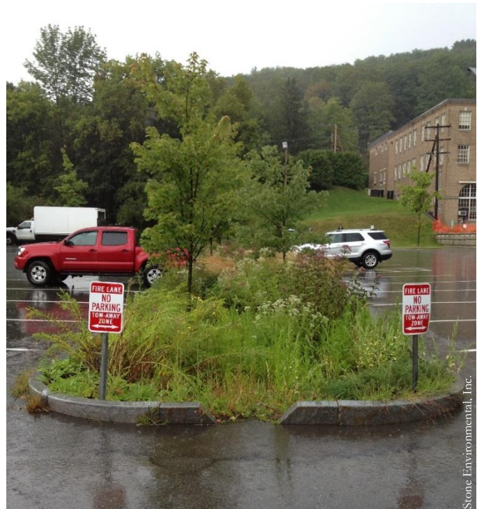
A dry swale in action during a rainstorm on State Street in Montpelier.
