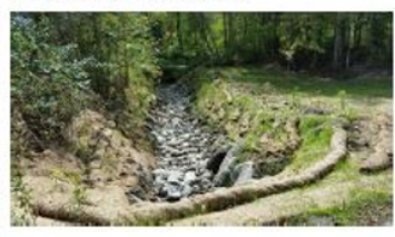
The restored gully on Depot Street after constructing and post-planting.
