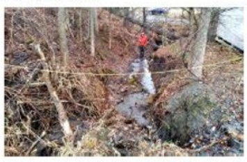
An eroded gully on Depot Street in Hyde Park before restoration.
