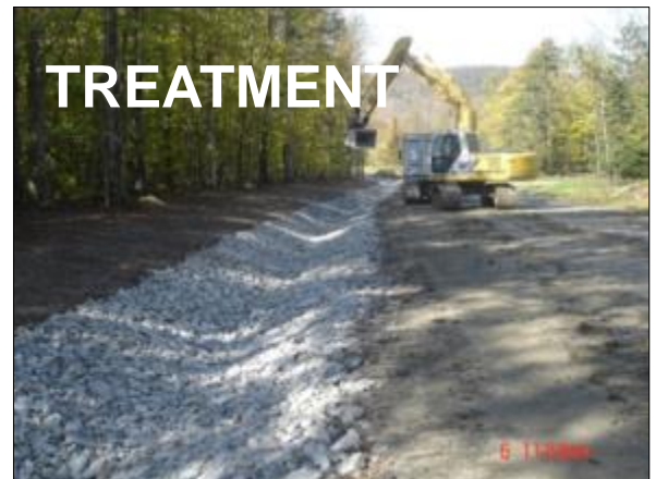
Ditch stabilization saves road and reduces erosion
