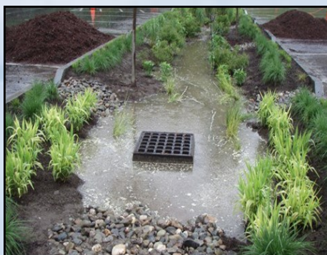
Green stormwater infrastructure receives
