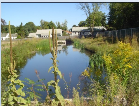
Expanded stormwater treatment pond
