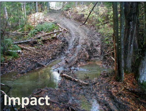
Poor stream crossing practice
