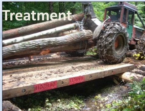
Portable skidder bridge protects water quality during timber harvesting
