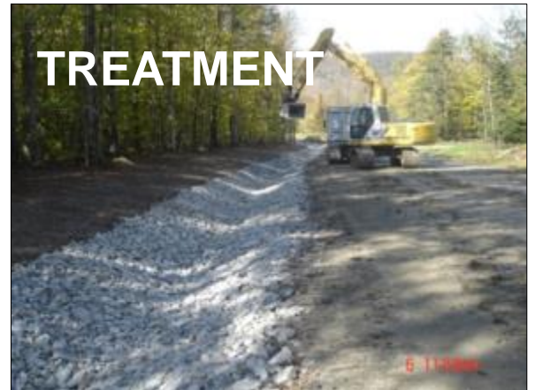
Ditch stabilization saves road and reduces erosion
