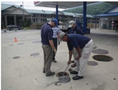
As of August 1, 2012, every permitted facility must have a designated A and B operator. **One of the more important responsibilities for the A/B operator is the monthly facility inspection requirement.** Routine facility inspections conducted by state inspectors reveal that some operators forget to perform and document their monthly inspections.
