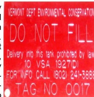
If a UST inspector finds a facility with dangerous compliance problems, or if owners/operators fail to conduct needed testing or maintenance, the UST Program may decide to affix Red Tags to the fill ports of the facility tank systems. The metal tags read "Do Not Fill", and serve to prevent deliveries to the facility. Needless to say, owners have been very quick to take necessary actions to return their UST system back to service.
