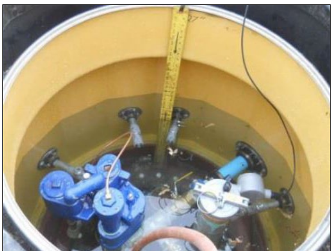
Figure 1: Conducting a hydrostatic test on a tank top sump.
