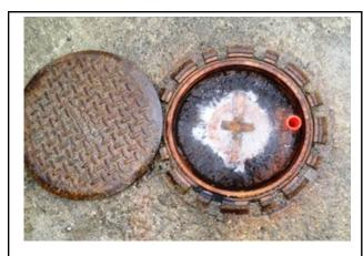
Our inspector found this spill bucket completely filled with ice. How do you suppose this tank owner will prepare for the next delivery?
