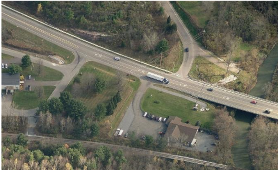
Laplatte River at RT 7 and rail line (site of DV-01b). Access road at left. View looks east.
