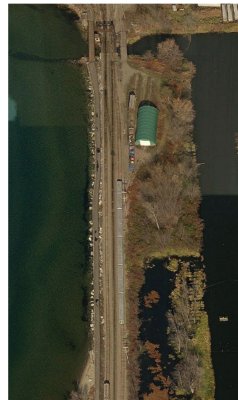
Aerial view of rail line leading into Vermont Railway Yard. Site of Containment Booming (C-02b).
