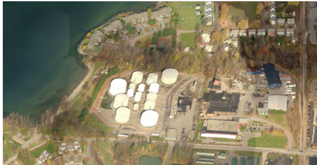
Site of EX-01e (left) near Global Partners LP Terminal.
