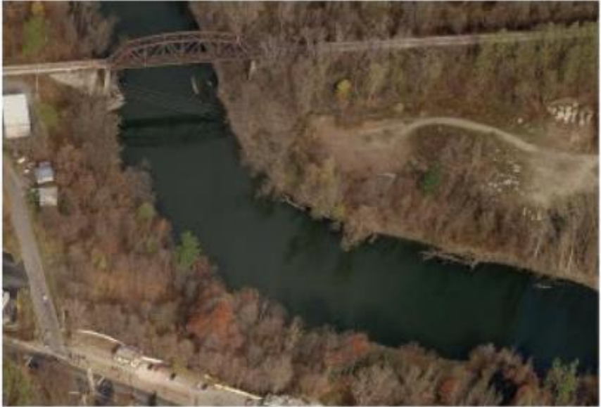
Site of DV-01b. View looks downstream.
