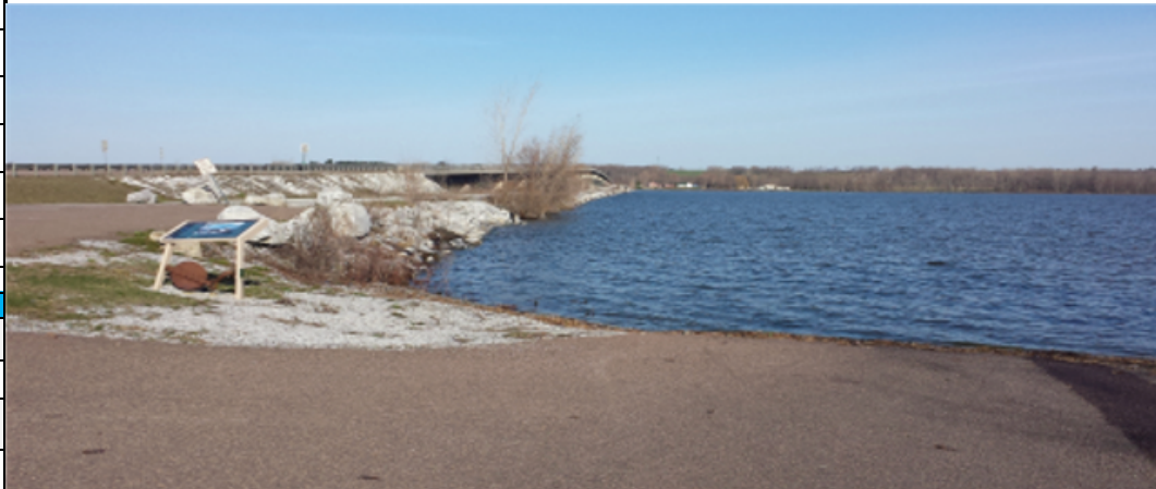
Route 78 bridge/jetty looking west from Larry Greene Fishing Access Area during Spring flood stage.
