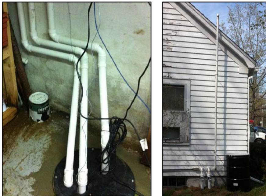
Sump remedial system under construction with two water discharge lines and one vent line (left); Sump air vent and discharge lines (right).
