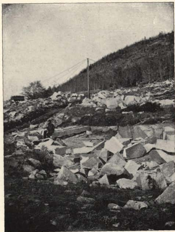
Blue Mountain Granite Quarry, Ryegate, Vt.
