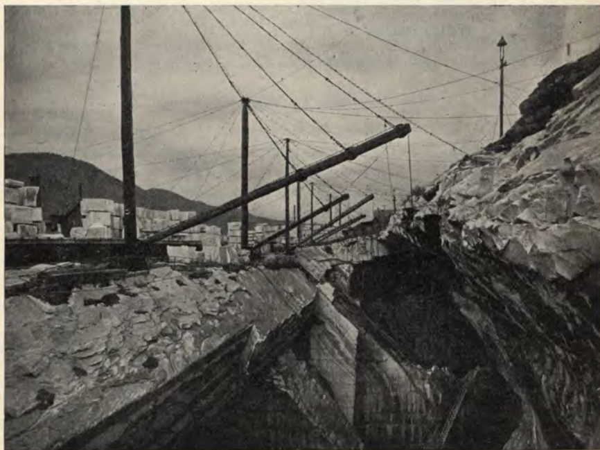
FIG. 19. East quarries at West Rutland.
