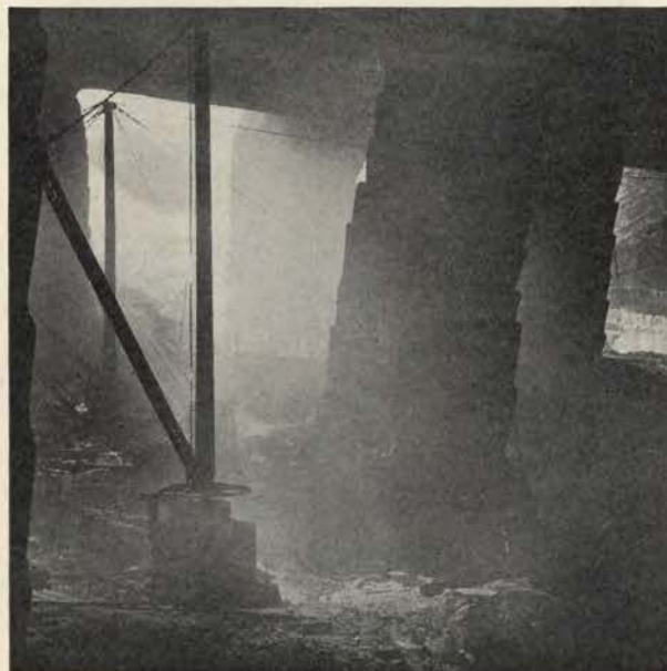
FIG. 21. Looking out from underground tunnels, West Rutland quarry.
