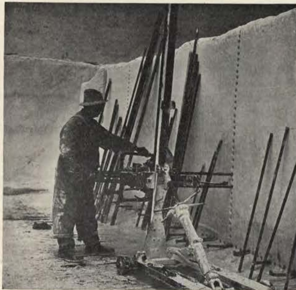
FIG. 40. Drilling in the marble quarry preparatory to wedging and splitting apart of the marble blocks.
