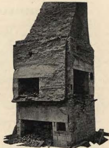
FIG. 4. Old Vermont chimney, after the house of wood has fallen away. Built 150 years ago and faced with marble slabs from Dorset quarries.
