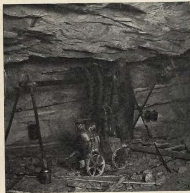
FIG. 10. Opening a new floor in the underground marble quarries.
