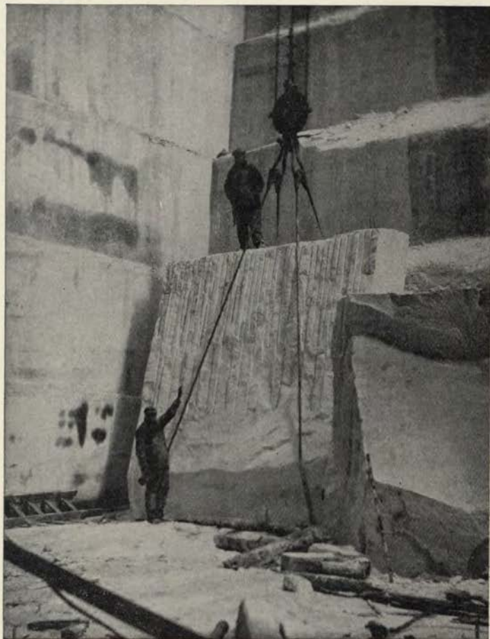
FIG. 13. Sixty-three ton marble block for bowl of Scott Memorial Fountain, Detroit, Mich.
