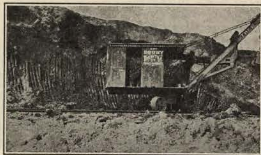
Thew automatic electric shovel.
