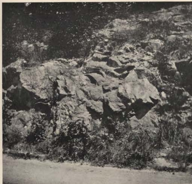
Outcrop of the Little Falls formation at Shoreham Center, Vt., showing its appearance in surface exposures.
