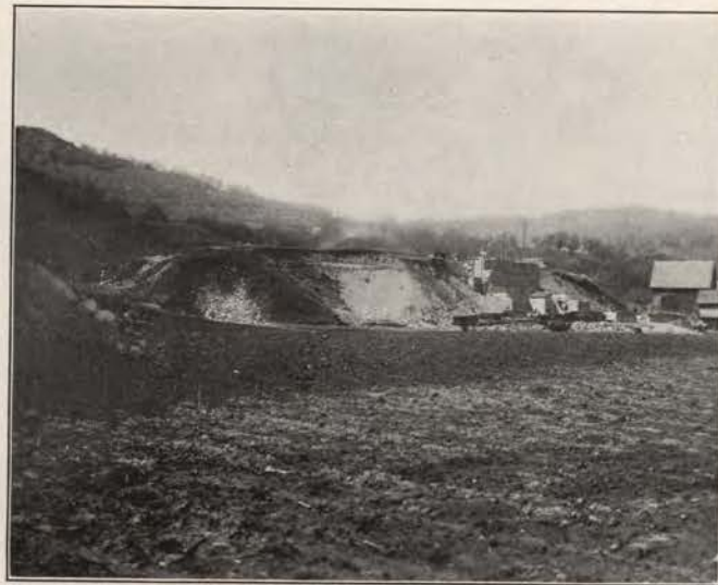
B. TERRACE EAST OF BRIDGEWATER.
