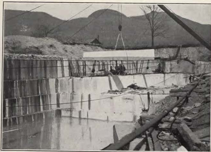
A. PART OF THE PLATEAU QUARRY AT SOUTH DORSET. Showing stripping and in the distance the Owl's Head and Green Peak. The block being hoisted is for a 32-foot column for the Art Building at Montreal. The black stains on the quarry walls are caused by the smoke of the cutting machines.
