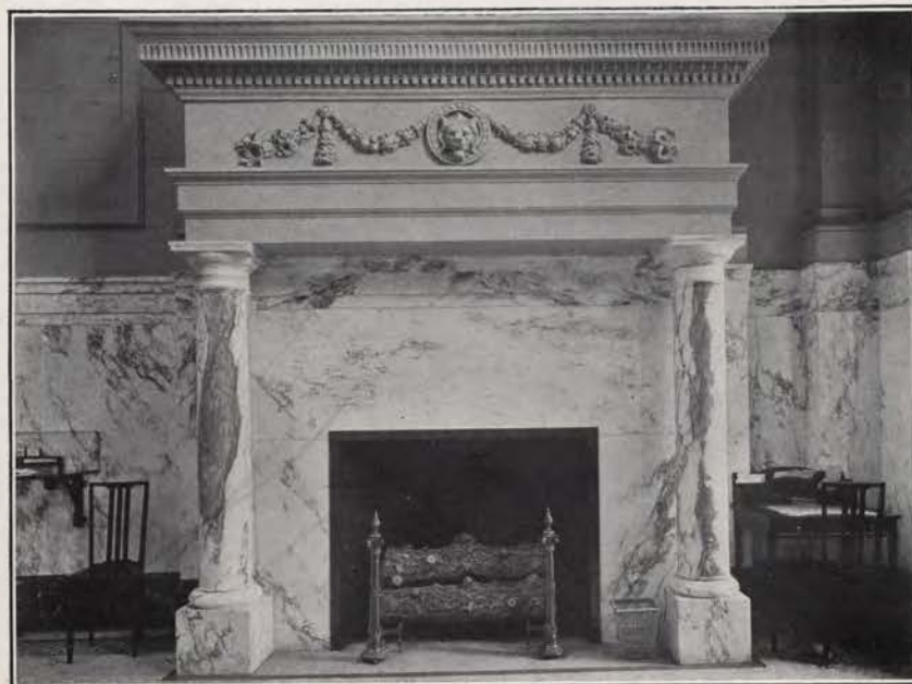
B. MANTEL AND WAINSCOTING IN FIRST NATIONAL BANK, HAZLETON, PA. Muscovitic calcite marble, "American pavonazzo," from West Rutland.
