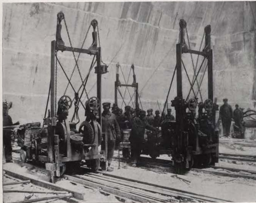
CHANNELING MACHINES AT WORK.
