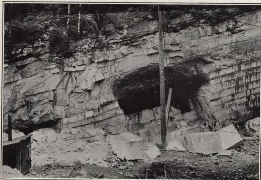
B. TUNNEL OF NEW YORK QUARRY, DORSET MOUNTAIN, DANBY, FROM THE NORTHEAST. Showing two sets of joints at the left of the tunnel due to a trap dike at the south (not shown in the picture). The marble at the tunnel and north of it is free from joints.
