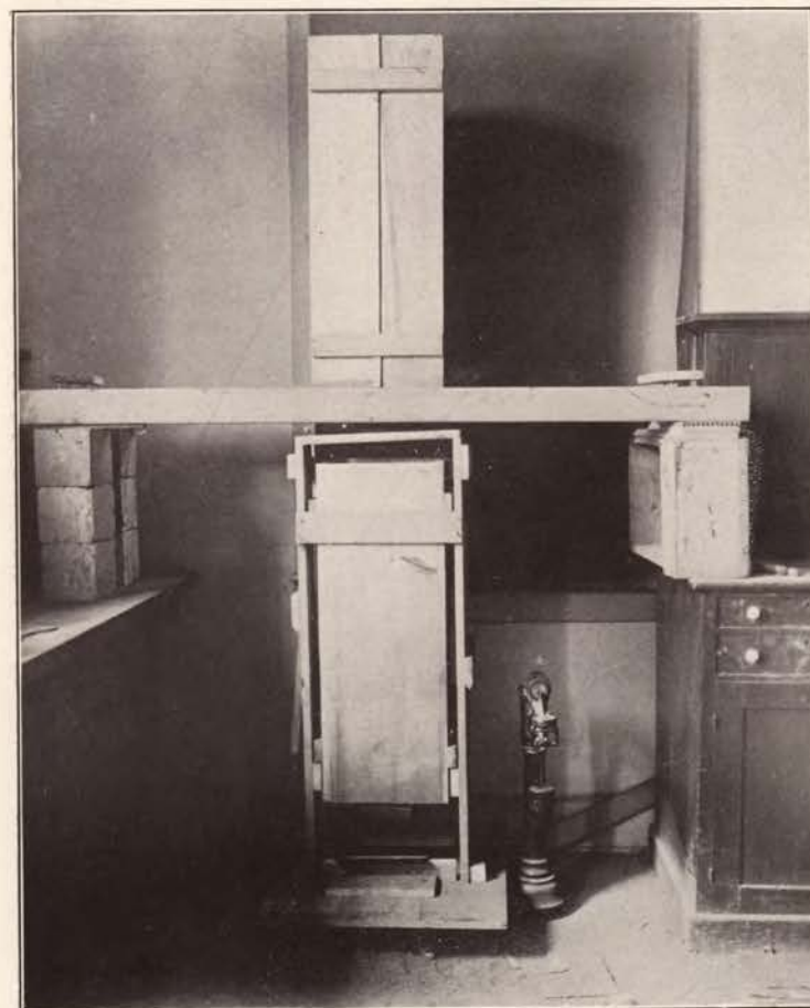
Apparatus for Testing Strength of Marble and Slate.
