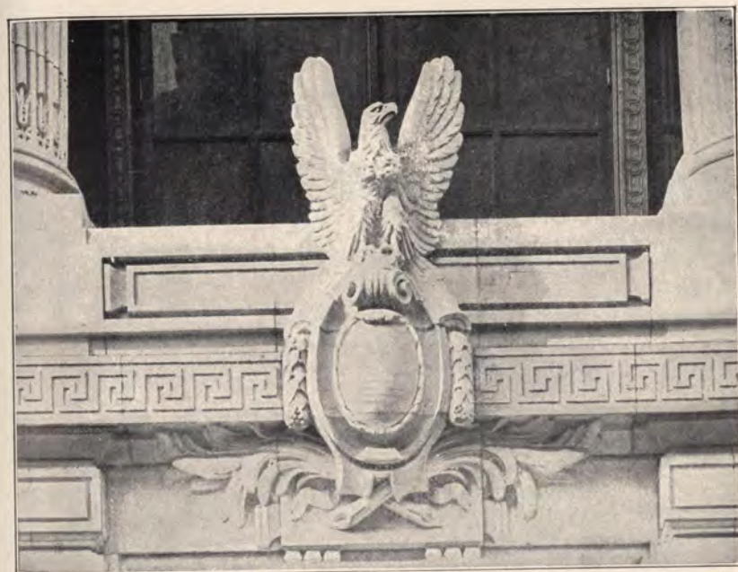
a. Carved Eagle of Coarse White Quartz Monzonite From Bethel Over Entrance to American Bank Note Company's Building, New York.
