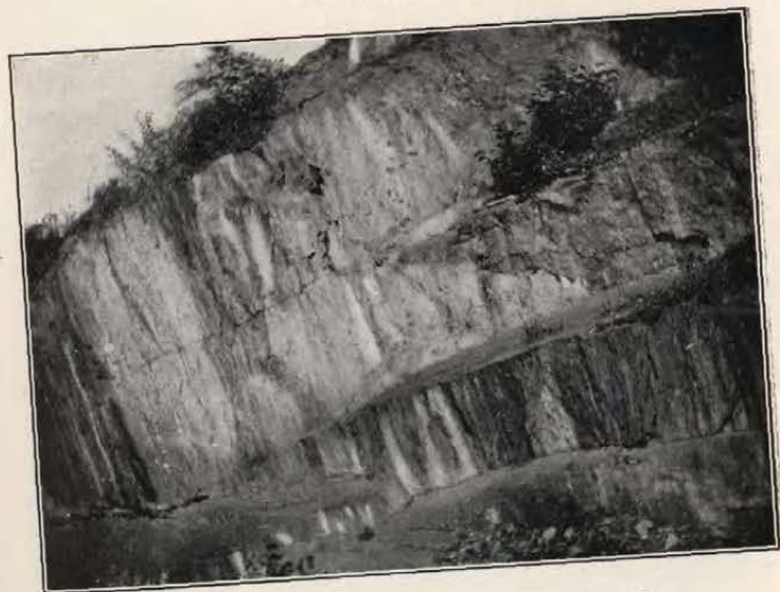
Railway Cut in Lunenburg Schist, Wells River, Vt.
