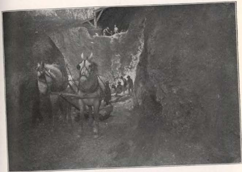
Looking into the Cut in Talc Mass.
