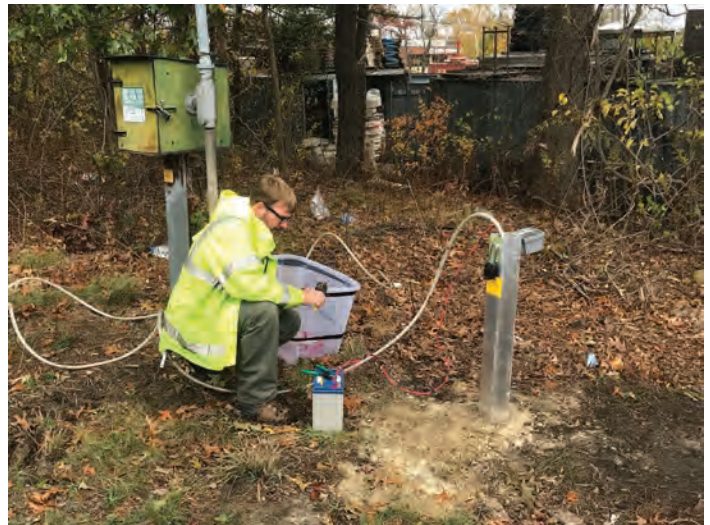
Figure 4. Developing the newly installed well in Wakefield, MA.
