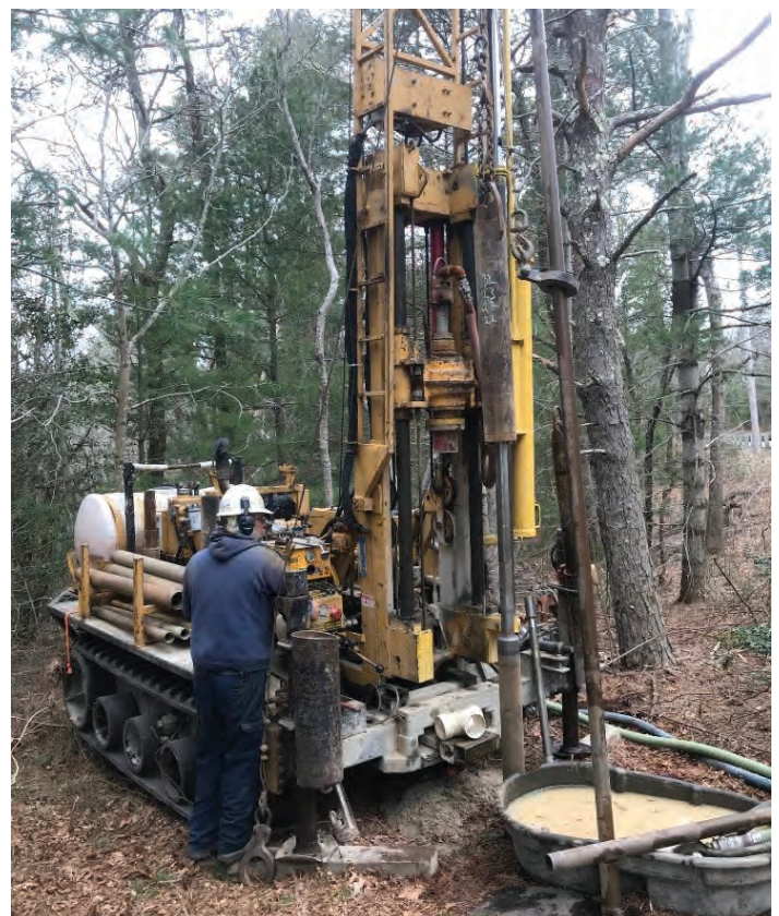
Figure 3. Drilling 70-foot replacement well on Cape Cod and installing 2-in. pvc casing.
