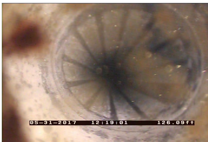
Figure 2. Well camera image of shallow coastal plain well as it approaches well screen.
