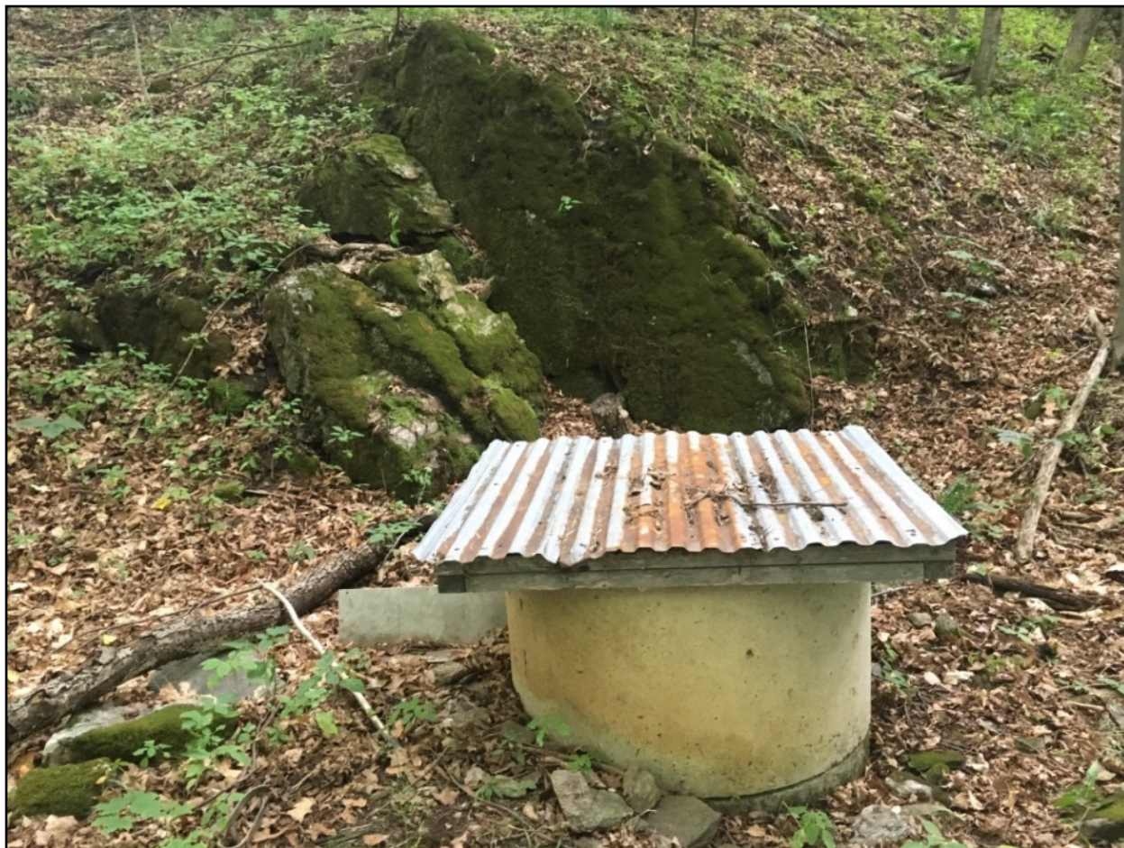
Figure 15: Shallow dug well in till adjacent to bedrock outcrop. Infiltration through the till is sufficient to supply water to shallow wells and to recharge the underlying bedrock aquifers.
