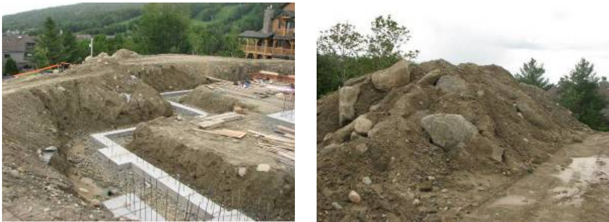
Figure 19: Exposure of dense till in Mt Snow Village development project illustrating less oxidation, higher clay content and larger clasts.
